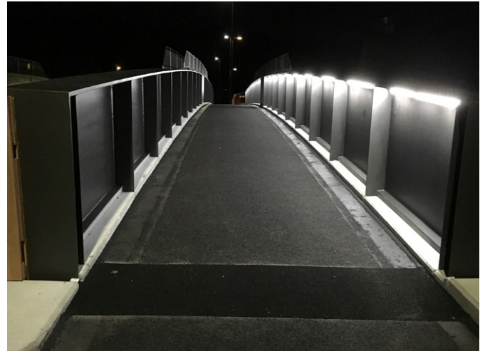
Pedestrian bridge Brügg
